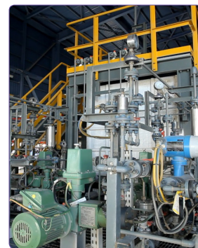
▲ UAE Oil Refinery Plant Chemical dosing system (120mL/day)
