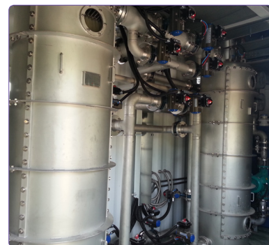
SK Innovation Petrochemical Reuse treatment system at petrochemical waste water (1,000m 3 /day)
