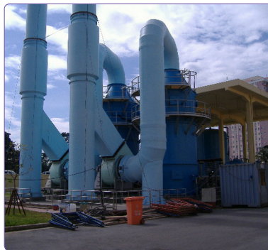
▲ Waste water treatment plant in HoChiMinh, Vietnam 3-stage liquid deodorizer tower (3,000CMM)
