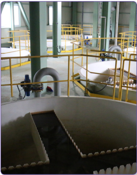
Kumho Petrochemical Gravity filter (16,800m 3 /day)
