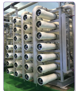
Jangmoon Natural Gas Power Plant Cooling water treatment system (5,900m 3 /day)
