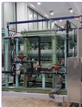
Shinboryeong combined cycle thermal power plant Seawater electro-hypochlorite system (1,200kg · Cl 2 /day)
