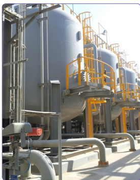
▲ Jubail Export Refinery in Saudi Arabia Condensate polisher (28,400m 3 /day)
