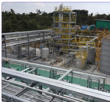
SK Materials Waste water treatment system (1,250m 3 /day)
