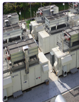
▲ Fuel cell plant Phosphoric Acid Fuel Cell
