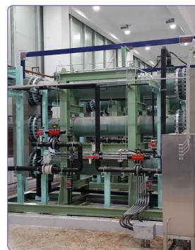
▲ Seawater electro- hypochlorite system
