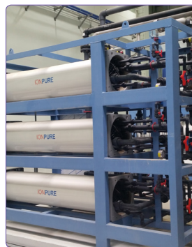
▲ Shinboryeong combined cycle thermal power Plant Electro-deionization (1,680m 3 /day)
