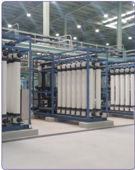
Shinboryeong combined cycle thermal power plant Ultra filtration (3,300m 3 /day)
