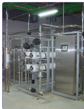
Dongwha Pharmaceutical Reverse osmosis & electro-deionization system (1,000m 3 /day)
