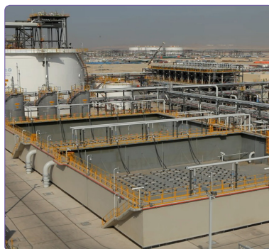
Ruwais Oil Refinery Plant in UAE Waste water treatment system at oil refinery plant (1,500m 3 /day)
