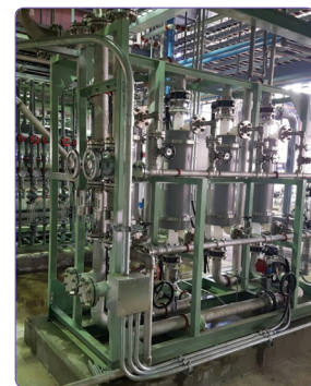
▲ Chuncheon combined cycle thermal power Plant Membrane deaerator (720m 3 /day)
