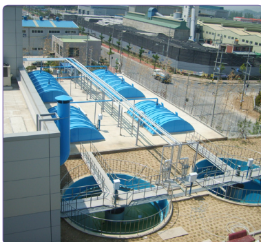
Yuhan Corporation Waste water treatment system at pharmaceutical plant (1,500m 3 /day)
