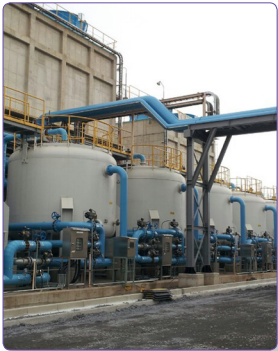
Hyundai Steel Pressure filter (6,800m 3 /day)
