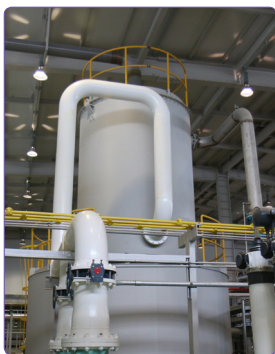
▲ Jangmoon Natural Gas Power Plant Cooling water treatment system (5,900m 3 /day)
